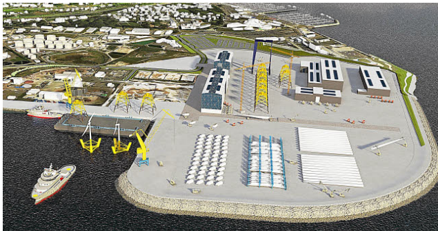
Work in progress for the construction of a polder in the port of Brest aimed at attracting activities related to marine energies
