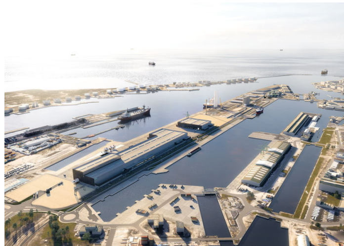
3D representation of the Siemens Gamesa Renewable Energy plant in Le Havre
